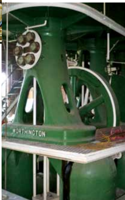
Steam-driven water pump installed in the late 1800s
