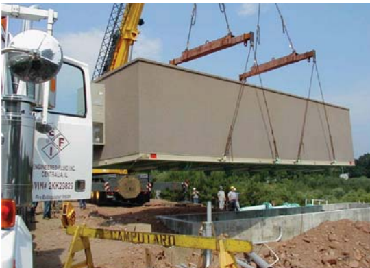
Off-loading enclosure from EFI truck with rigging supplied by EFI.
